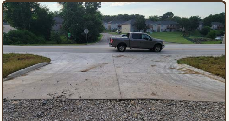
New concrete entrance off Highway 76
